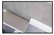
Installation of insulation panels with double buttering
