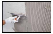
Installation of insulation panels with double buttering (on wall)
