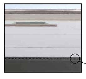
The special, patented CeraVent<sup>®</sup> matting **CeraVent**<sup>®</sup> favours drainage, ventilation and decoupling.
